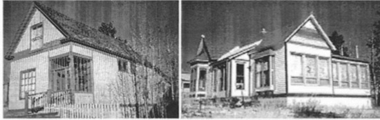
Historic additions were in the rear, and "stepped down" in scale from the original house.
